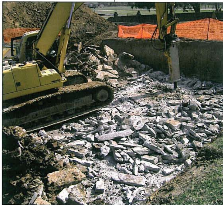
A hoe ram breaks up two feet of limestone before laying a 12-inch gravel base for the last four biofilters.
