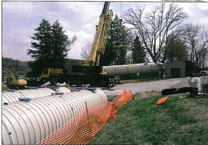
Outriggers support a 200-ton crane as it lifts a 15,000-pound EnviroFilter biofilter tank and prepares to set it 90 feet away on a gravel bed.
